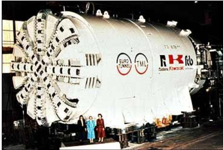
*A photo of one of the tunnel borers used for the Chunnel in 1985. This borer was just under 29 feet in diameter. In contrast the borers to be used in the peripheral tunnel will be four feet GREATER in diameter, 33 feet total. The cost of the Chunnel was 21 billion in 1985 money. The peripheral canal tunnels will be almost twice as long and four more feet in diameter but the "guesstimate" for the cost is similar to the cost of the Chunnel, 21 billion. Really?*
