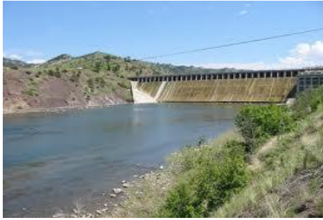
Holter Dam on the Missouri. Photo courtesy of BigSkyFishing.Com
