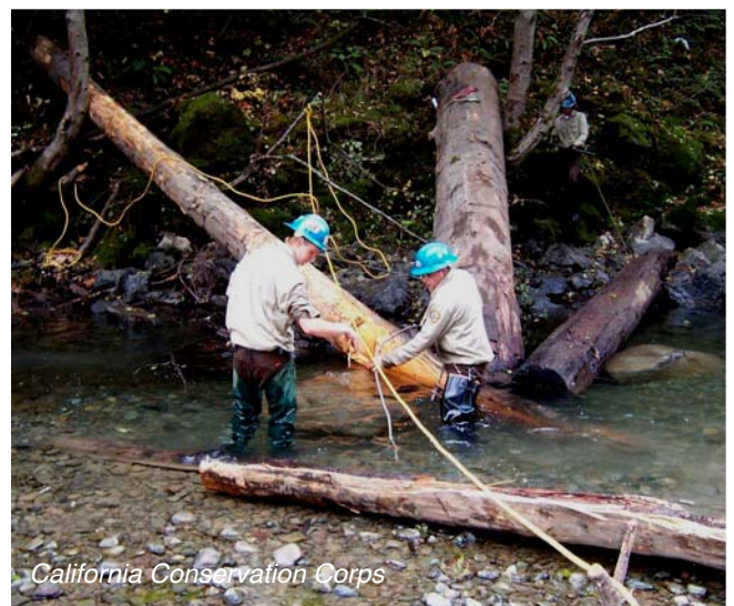
CCC crew installing large woody debris
