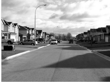
Suburban style, no sidewalks
