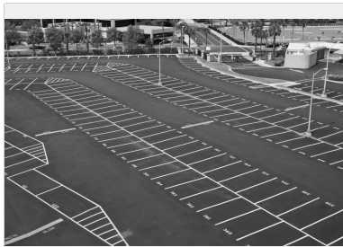
Asphalt paving with lighting
