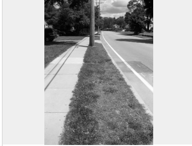
Sidewalk with grass landscaping
