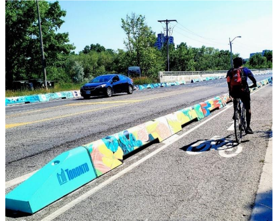
An example of a quick build project is a cycle track that includes concrete barriers.
