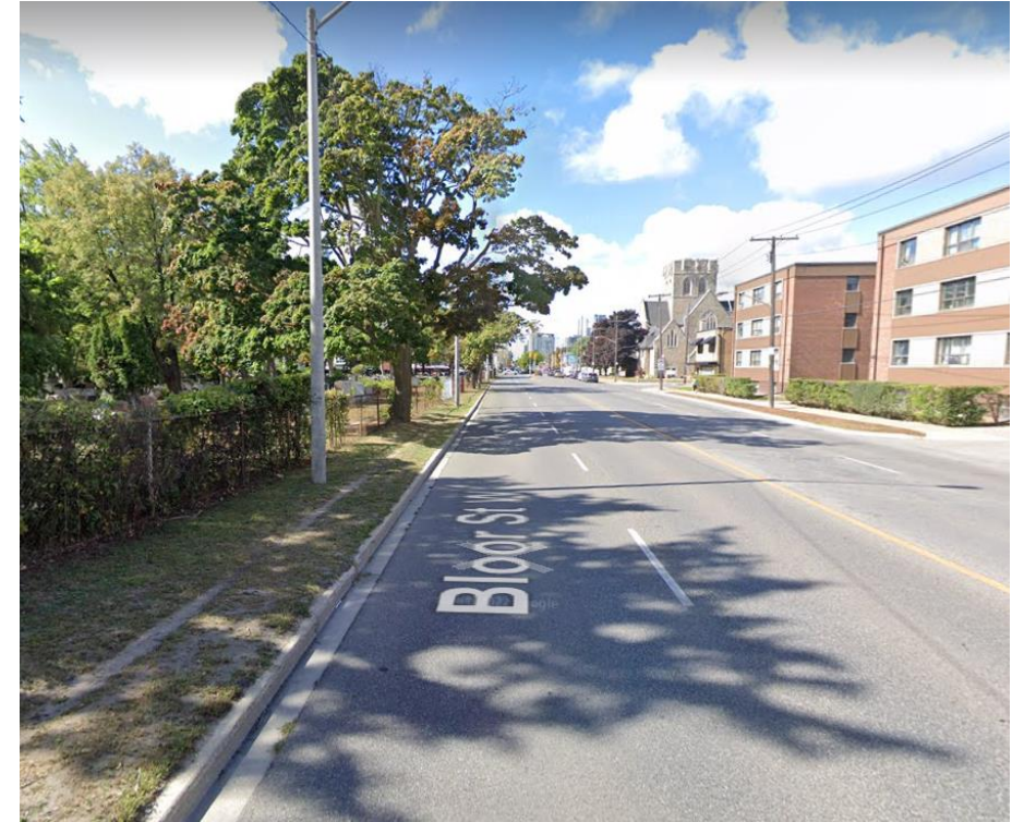
Sidewalk gap Between Prince Edward Drive and Kingscourt Drive (south side)
