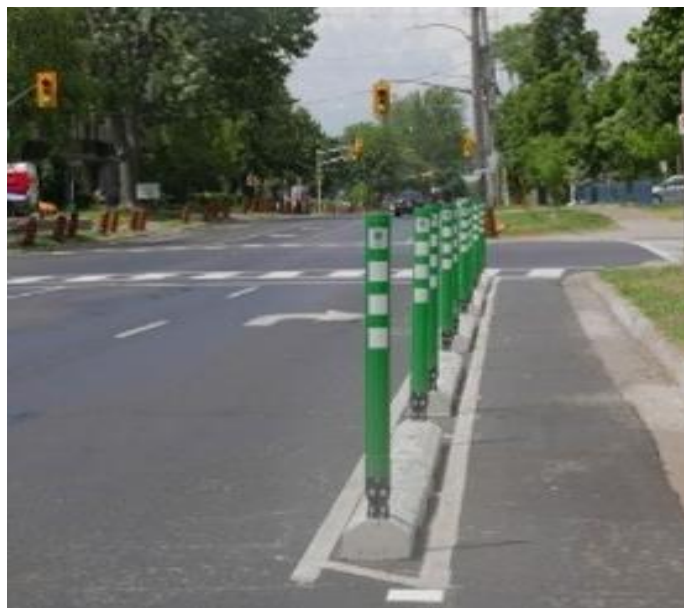
Flexible Bollards on Pre-cast Concrete Curbs
