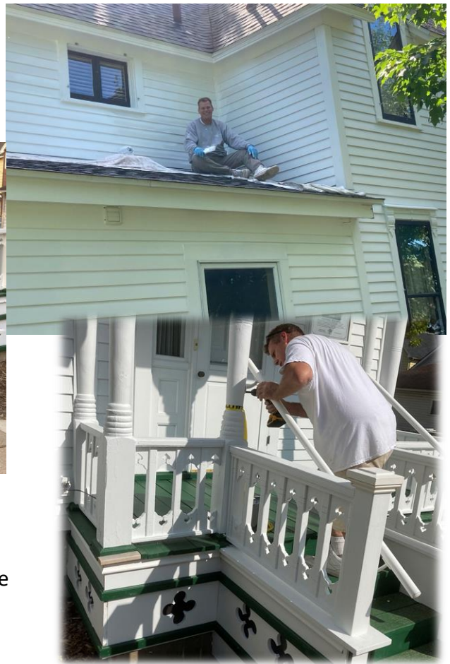
And the carpenter/painter paints
