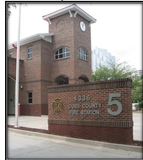
Cobb County Fire Station #5
