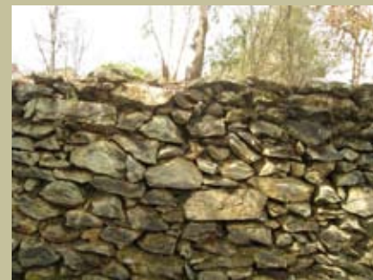
DRY STACKED ROCK WALL
