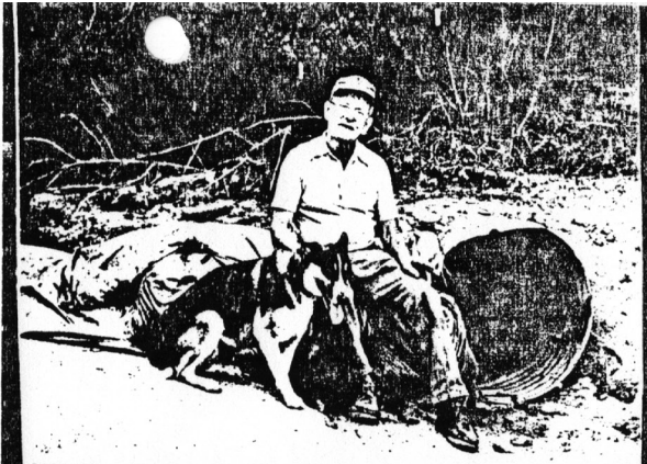
RESTING — DeLuz rancher Felix Garnsey takes a breather beside a culvert he had to shore up recently with sand in plastic garbage bags to stop water from washing out the culvert. Garnsey found that using plastic to cover loose soil greatly restricted the water's cutting edge.
