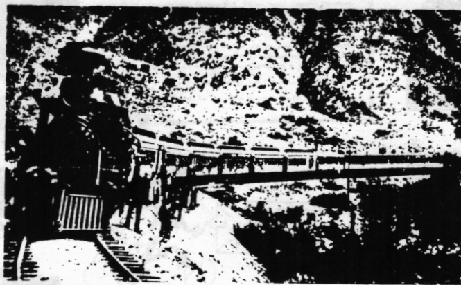
When the California Southern Railway was completed from San Diego to Temecula, excursions were run frequently. This old photo shows an excursion train, stopped in the Temecula or Santa Margarita Canyon not far from De Luz Station. The tracks were washed out in 1884, and again in 1891, and never rebuilt after the second flood.
