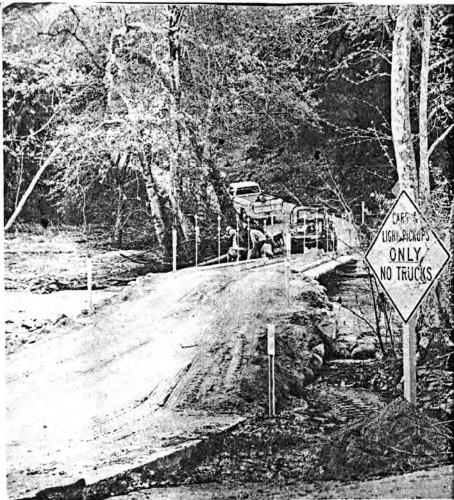
NEW CROSSING — Only cars and light pickups are being allowed to cross DeLuz Creek on the new steel bridge put in place by the department of transportation last week. The structure was being used temporarily until the water in the river lowers and a permanent bridge can be built to replace the one washed out two weeks ago.
