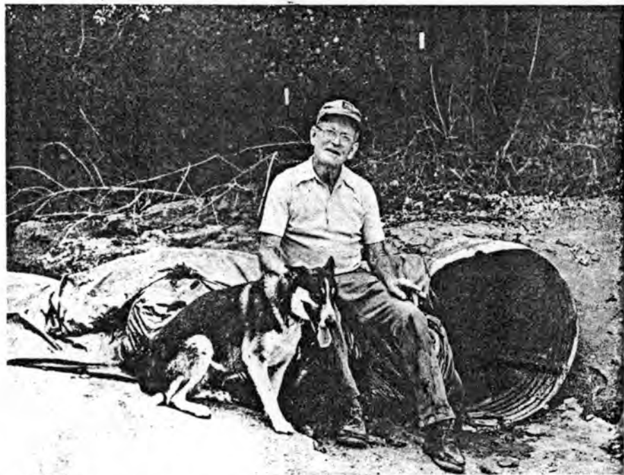
RESTING — DeLuz rancher Felix Garnsey takes a breather beside a culvert he had to shore up recently with sand in plastic garbage bags to stop water from washing out the culvert. Garnsey found that using plastic to cover loose soil greatly restricted the water's cutting edge.
