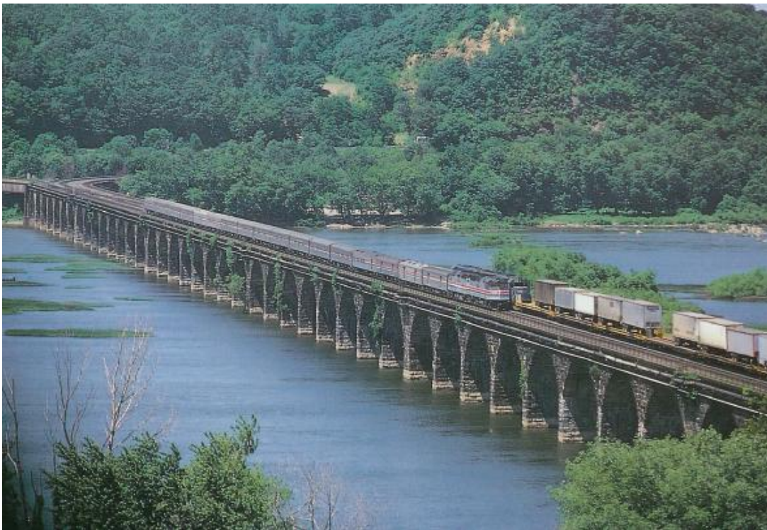
The Rockville bridge in Harrisburg was constructed and completed in 1902 by the Pennsylvania railroad. It took 800 workers 2 years to build. It is constructed
