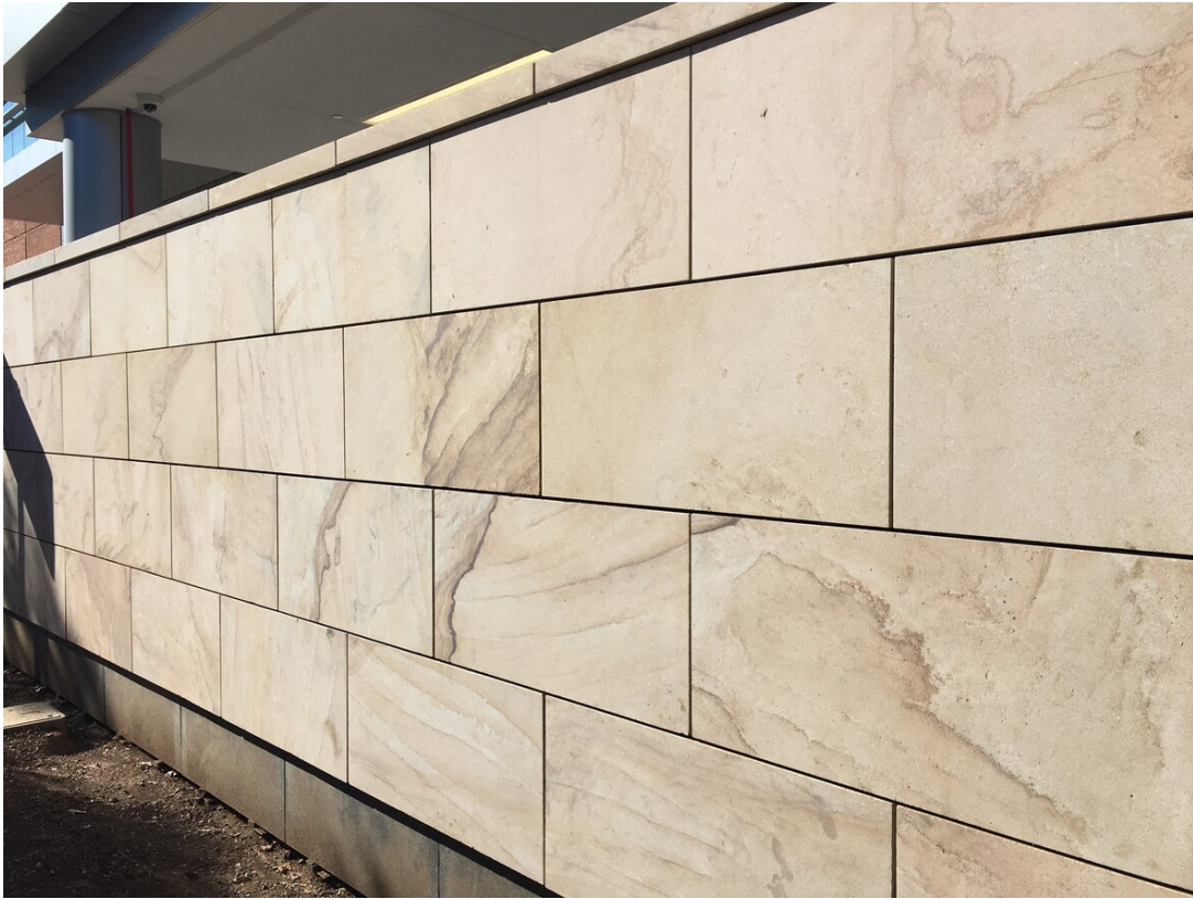
Retaining walls for large and smaller projects.
