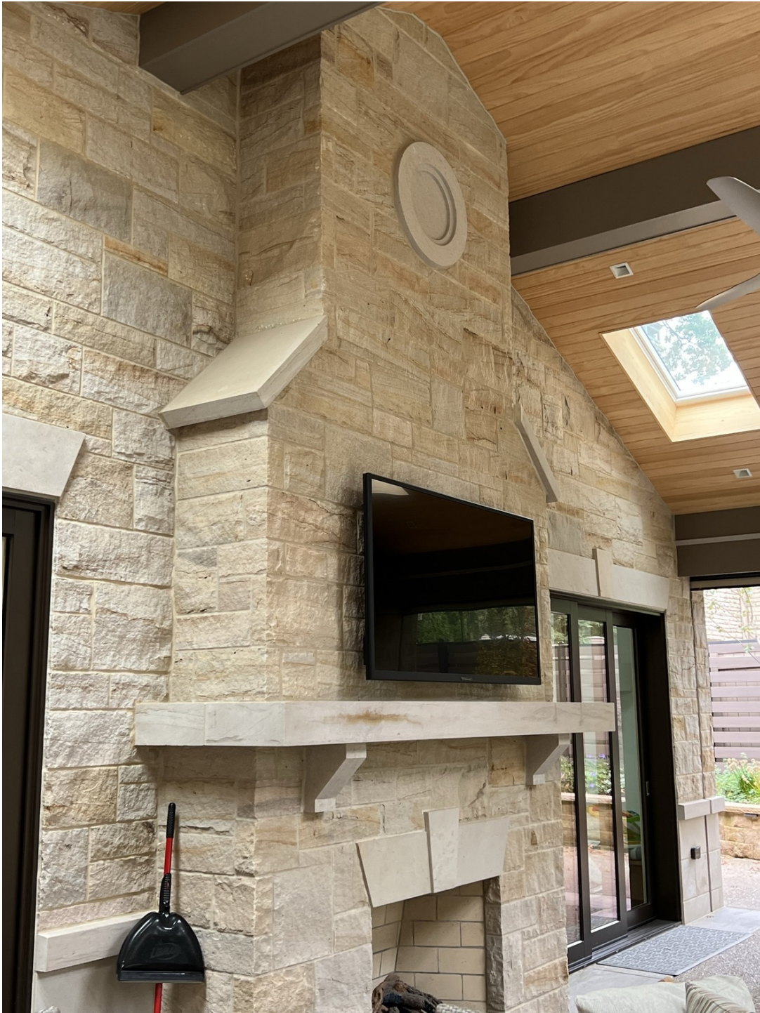
The stone used on the residence was a combination of stone panels and sawn bed building stone, sawn on 4 sides with hand rock faced fronts.
