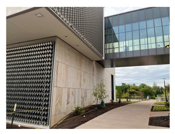
We provided panels of our Class II Approved Roaring Run Sandstone for the exterior of the project. The honed panels were 2" thick ,16" wide, and ranged in length from 2 to 5 feet. The design concept was to clad the building in regional sandstone evoking the geology of central Pennsylvania.
