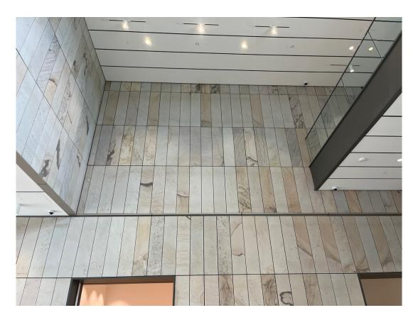
Several locations on the interior of the building also utilized our sandstone. We provided approximately 3800 square feet in panels that were 1 1/2" thick, 16" wide, and from 2 to 5 feet in length.
