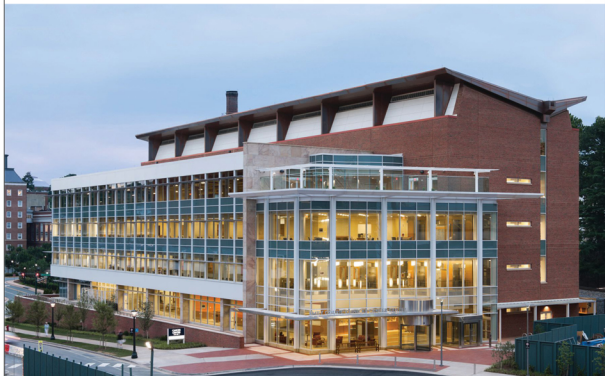
Select Oak Run sandstone was employed for various exterior and interior applications of the Emily Cosovic Clinical Cancer Center for the University of Virginia Health System in Charlottesville, VA. All photos by Chuck Choi Architectural Photography / www.chuckchoi.com
