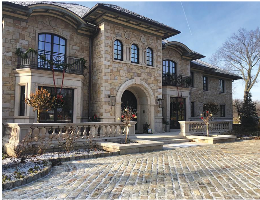
The lighter color of the material, which is Roaring Run Stone from Russell Stone Products, was appealing to the homeowners.
