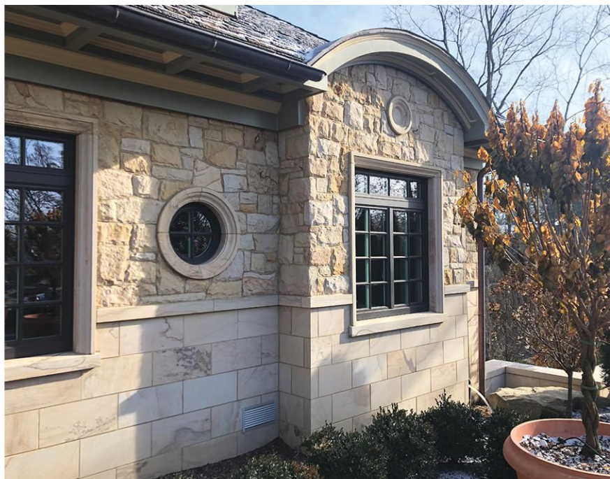
The stone was employed in both smooth and rockface finishes, which provide a nice contrast and texture to the exterior design.
