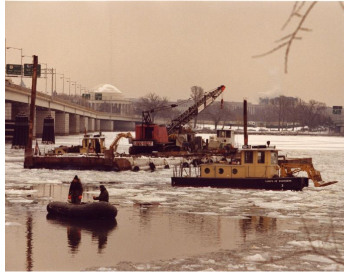
Photo of BD-5 taken during Air Florida 90 recovery efforts in January, 1982. (US Army Corps of Engineers photo)
