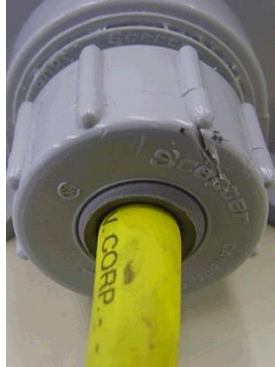
strain relief connector/compression fitting showing flexible cord entry
