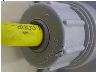
Flexible cord with a compression type strain relief
