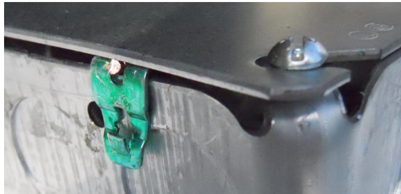
Exterior view of box with cover in place-notice that the clip is visible You can see the cover does not fit/seat tightly against the box
