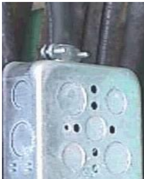
Romex type box connector improperly used on flexible cord and UL listing instructions and use of connector indicated on packaging
