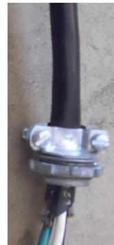
Romex type box connector improperly used on flexible cord and UL listing instructions and use of connector indicated on packaging
