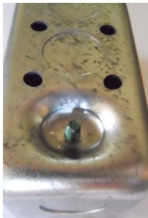
Screw visible through rear of box
