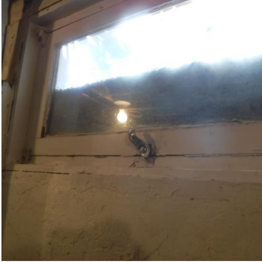
Basement window below grade-no wells
