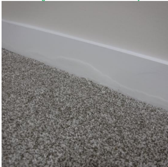
Moisture staining on ack wall in basement
