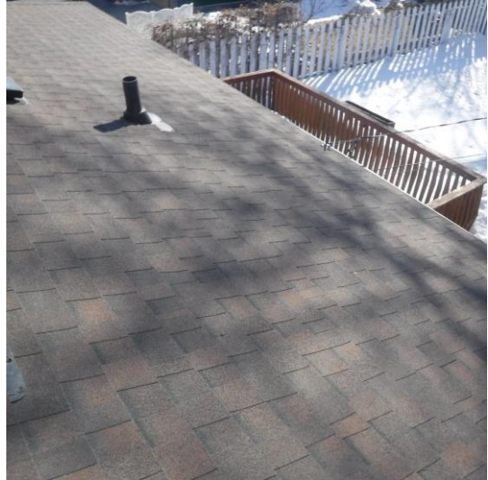
Shingles at back
