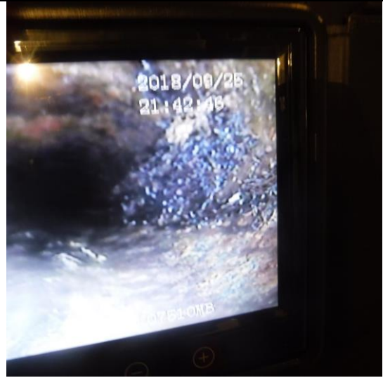
Roost in cats iron line in basement slab
