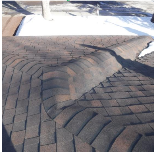
House shingles at front
