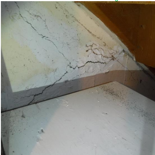
Cracking/inward movement in west foundation wall
