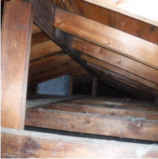
Roof structure in attic
