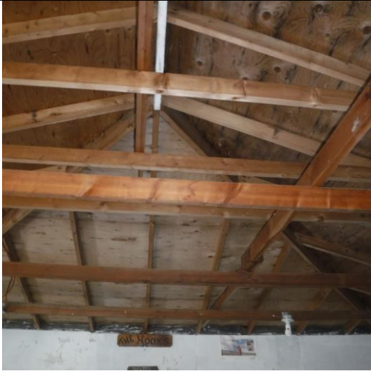
Garage roof structure
