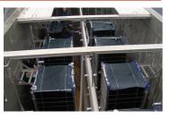
The STEP-MBR combines the principle of extended aeration activated sludge process with superior liquid/solid separation using gravity flux hollow sheet membrane modules. The STEP-MBR is one of the most simple MBR product on the market while achieving pristine effluent quality compatible with the most sensitive areas.
