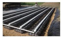
ELJEN GSF modular geotextile biofilter combined with a sand filtration system developed by Eljen Corporation and distributed by Enviro-STEP Technologies. ELJEN GSF is 100% passive. No electricity. No mechanical parts.
