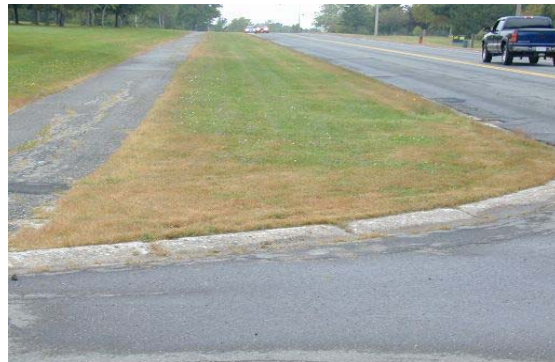
Figure 2-6. The results of capillary barriers introduced during construction.
