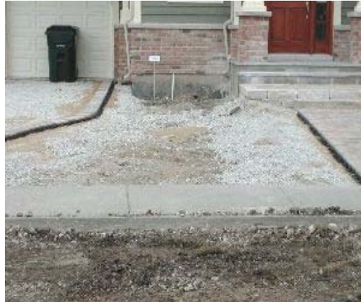
Figure 2-5. Construction sites with concrete (left) and crushed rock (right) about to be covered with soil, creating a barrier to capillary moisture movement. Photos courtesy of Dan Dinelli.
