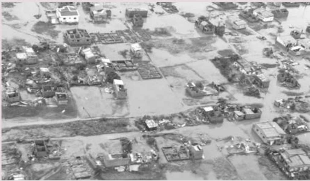
Destruction from Cyclone Idai in southeast Africa
