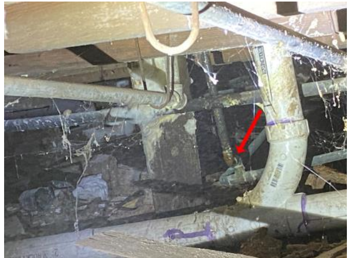
Leaking Pipe
