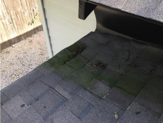
Low lying area on the roof
