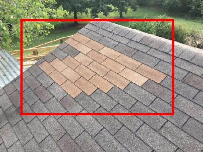
Repairs made to the area
