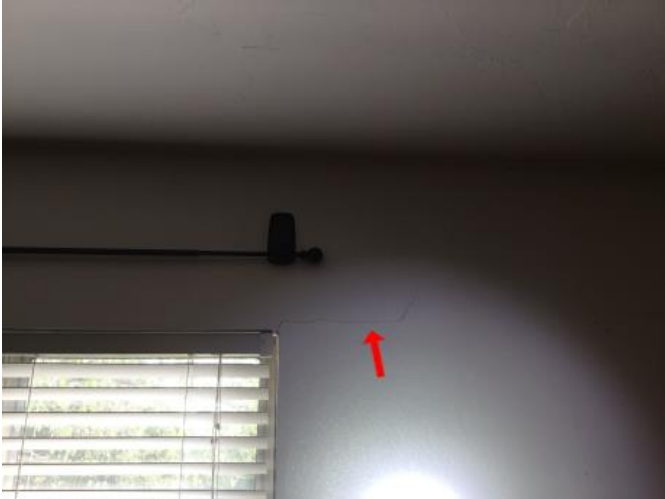
Settlement Crack
