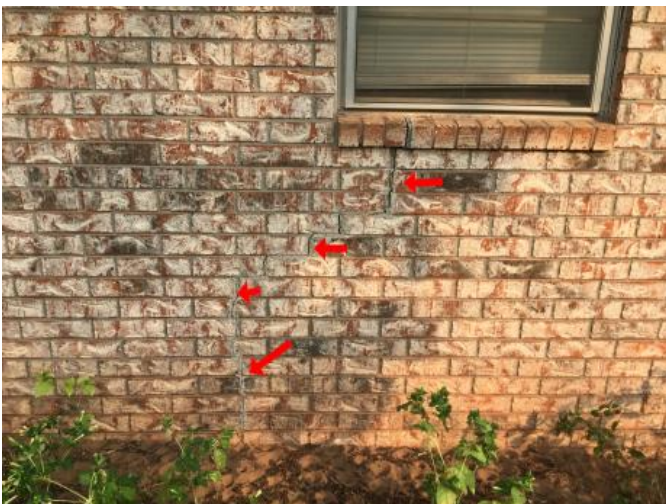
Settlement Crack
