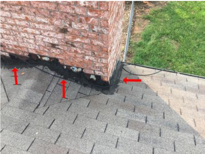
Chimney flashing repaired with roofing sealant
