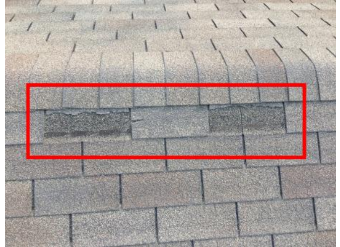
Broken Shingles
