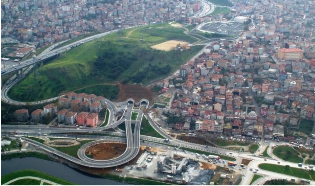
7 TEPE-7TÜNEL PROJECT, KAĞITHANE EXIT INTERCHANGE PROJECT - ISTANBUL March-2009
