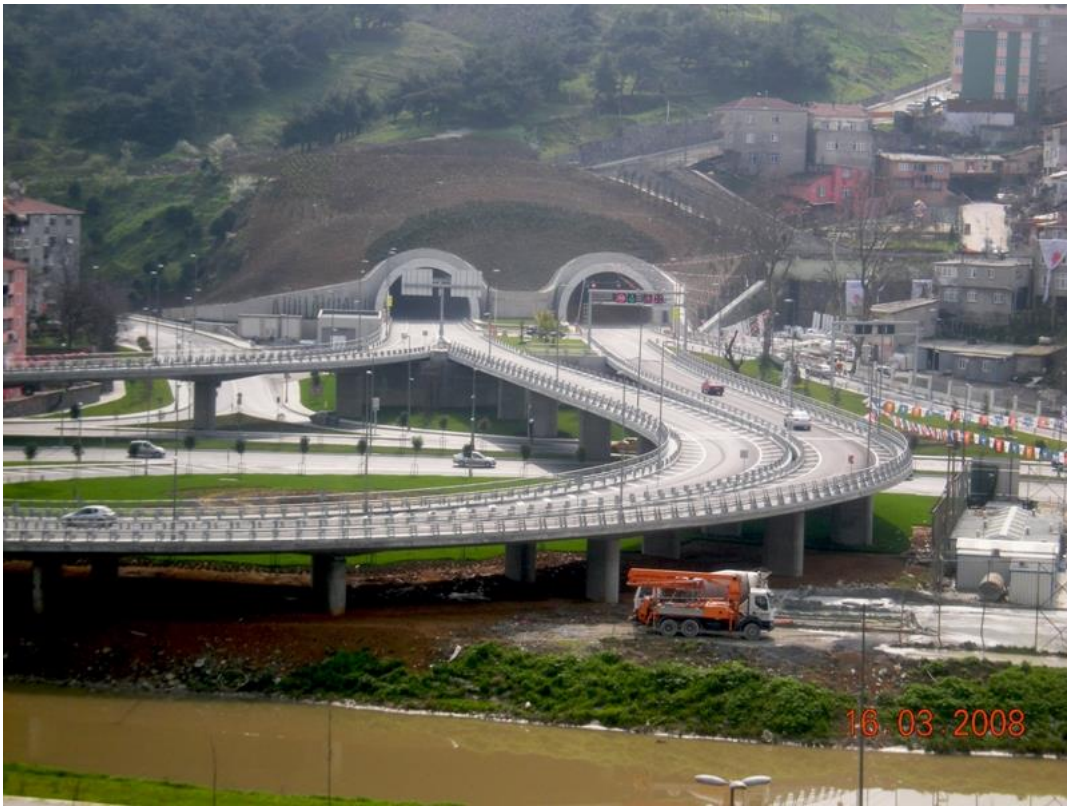
7 TEPE - 7TÜNEL PROJECT KAĞITHANE EXIT INTERCHANGE PROJECT - ISTANBUL March-2009
