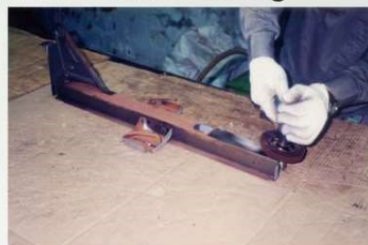
除銹中 In de-rusting
