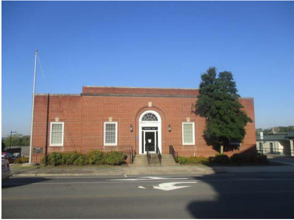
View of the front of the building.
