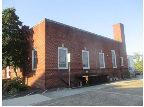
View of the northerly side of the building.
