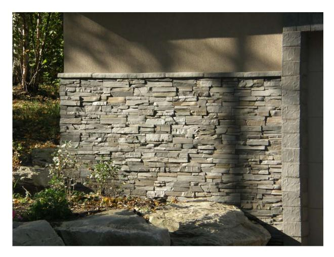
The lightweight stone was attached to the expanded polystyrene (EPS) substrate using our proprietary, polymer-modified cement plaster, which was also used as the basecoat over the EPS board. This formed the undercoat for both the stone and the beige acrylic stucco finish shown above the stone section of the walls.
