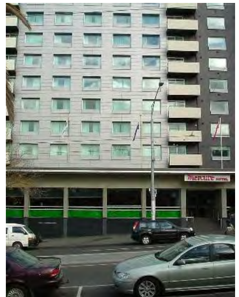
Office arcade street frontage treatment
