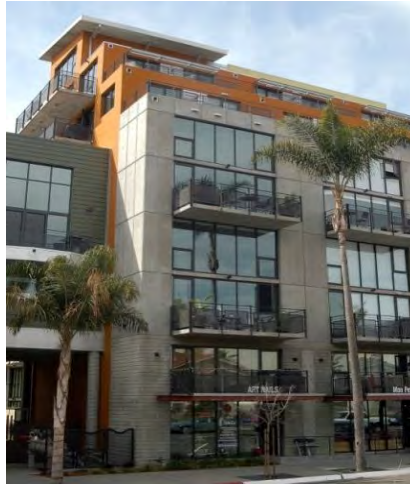
Varying building roof heights provide opportunities for roof terraces and help break building mass
