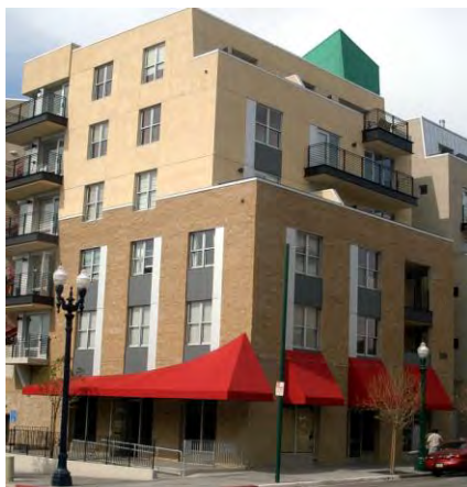
Awnings help make building access points more prominent and can help create a visually attractive contrast on a building façade
