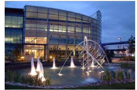
Office development clustered around common open spaces and sidewalks
