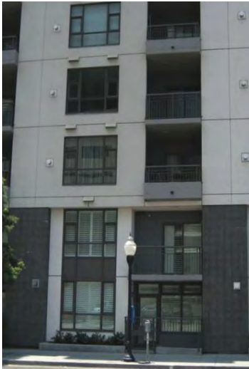
Base treatment may extend up to the top of the second level on buildings that are four stories or higher
