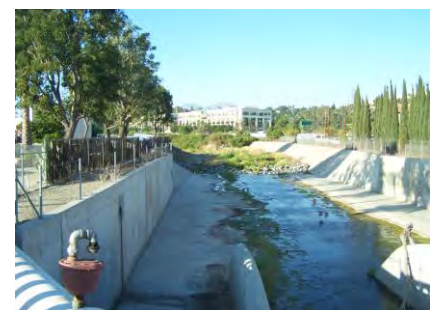
Oso Creek drainage channel
