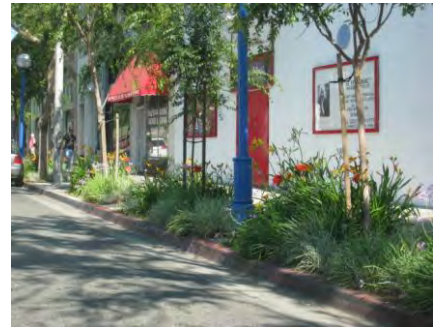
All continuous landscaped parkways collect stormwater runoff from the sidewalk
