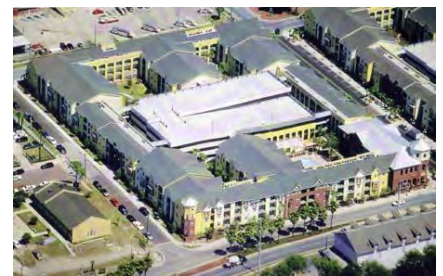
Wrapped Block building structure with double loaded buildings arranged around a central parking structure and courtyard open spaces
