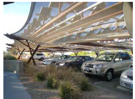
Photovoltaic panels may be incorporated into the roof of parking structures or over surface parking
