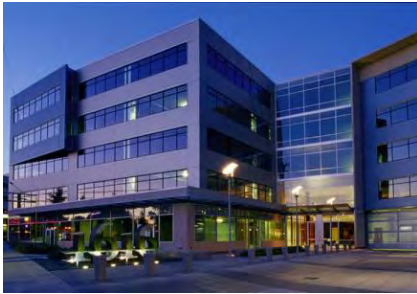
Offices oriented to the street
