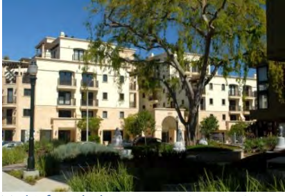
Multi-family housing (80 units/acre)
