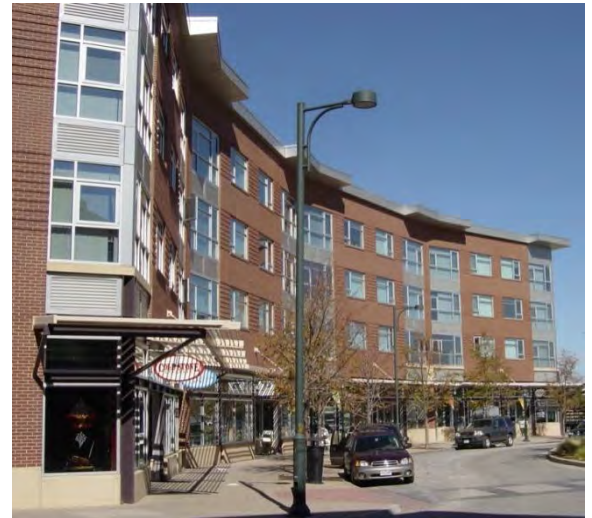
Thicker base portion and continuous awning element create a pedestrian-scaled ground level façade in this retail/office Mixed-Use building
