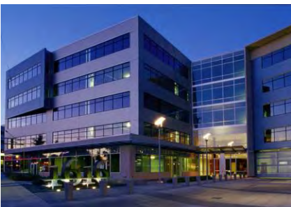
Office building showing a protruding horizontal shelter base treatment element at ground level
