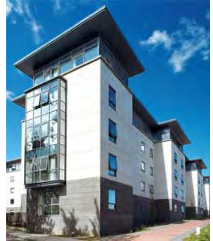
Contemporary style office building with precast concrete as a base treatment on ground level
