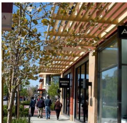
Ground level trellises add shelter and create pedestrian scale along front façades
