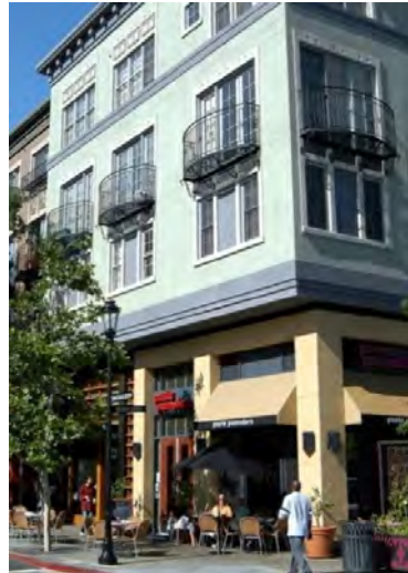
Ground level minor recess base treatment
