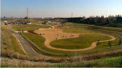
Joint use of storm detention facility (Sacramento, CA)
