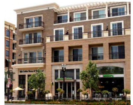
Mixed-Use building with upper-story window-to-wall ratio that is lower than the ground floor
