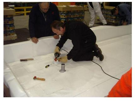
PVC Deck, Proper Welding Procedure for Repairs.
