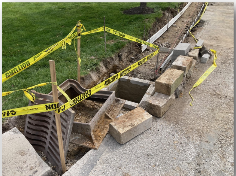
Storm sewer under repair and finished product
