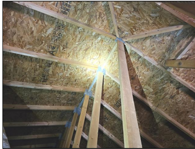
Roof Sheathing Material
