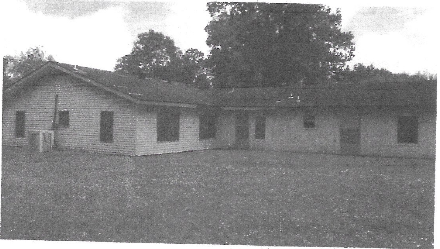
REAR VIEW OF RESIDENCE
