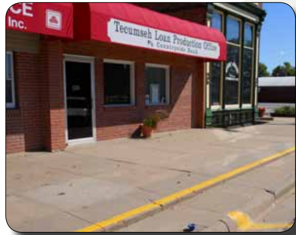
EXISTING BUILDING FAÇADE
