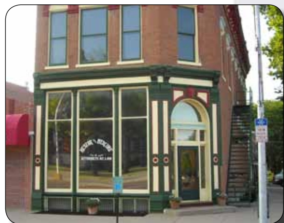
EXISTING BUILDING FAÇADE
