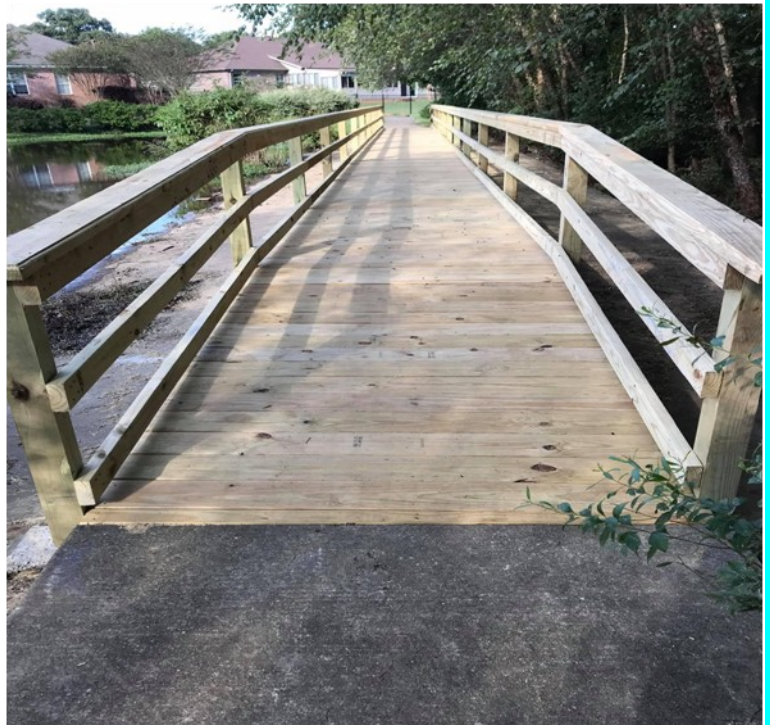
The Bridge has been treated with preservative
