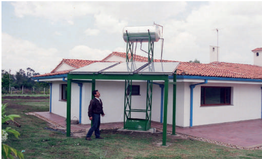
GAVIOTAS solar heaters installation in rural area Tenjo
