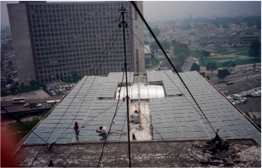
GAVIOTAS solar water heaters installation in Mederi Hospital Bogota
