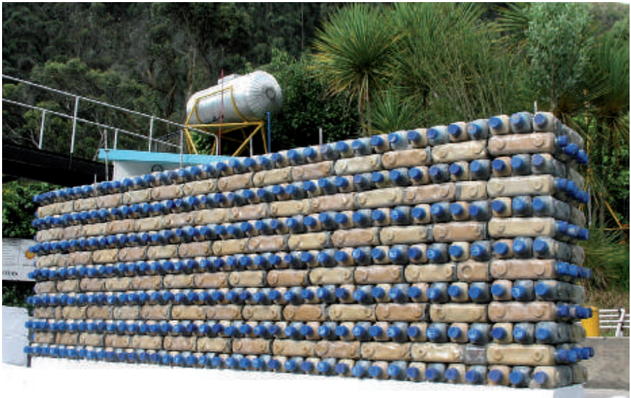
Recycling water bottles for GAVIOTAS housing wall construction
