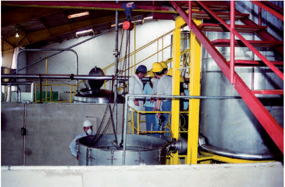
Partial aspect of arboquímica biofactory, GAVIOTAS
