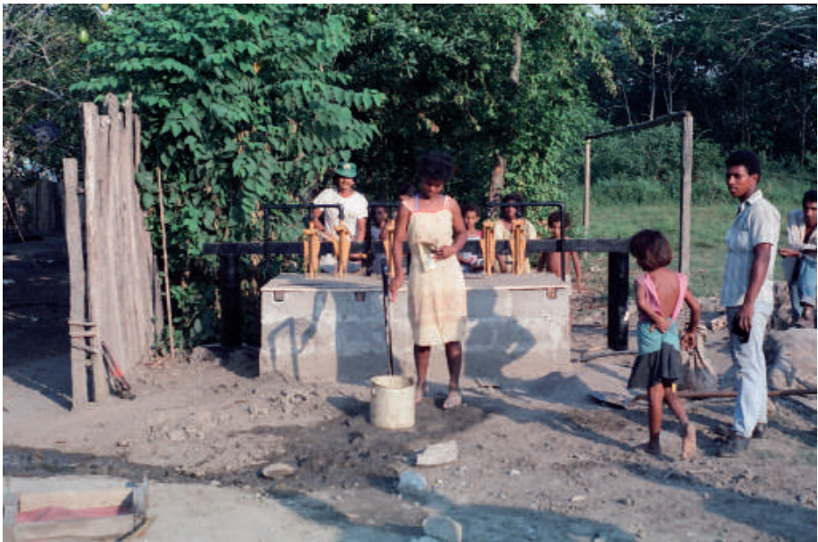
GAVIOTAS micro-acueduct with sleeve water pumps
