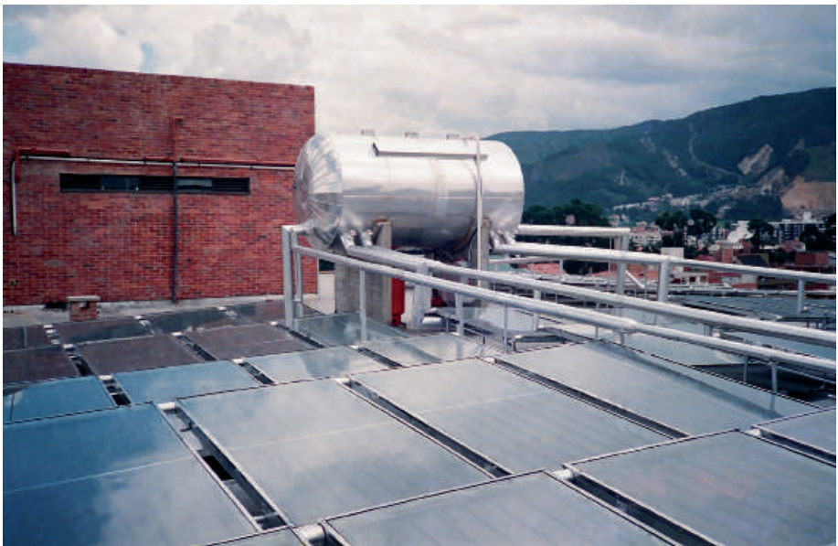
GAVIOTAS solar heaters installation in a Bogota Hotel
