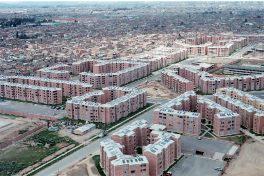
GAVIOTAS solar heaters installation in Ciudad Tunal, the biggest in the world in Bogota
