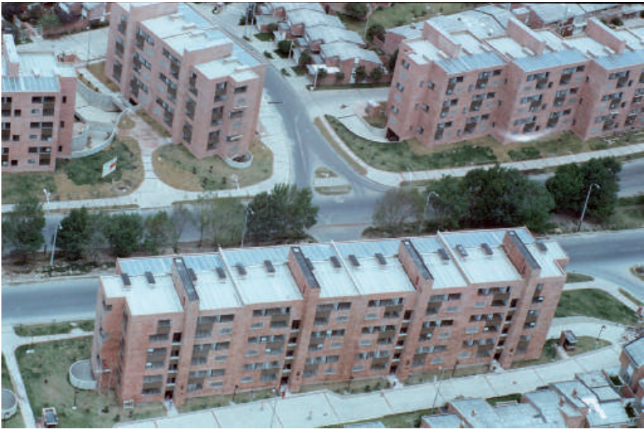
GAVIOTAS solar heaters installation in Niza VIII Bogota
