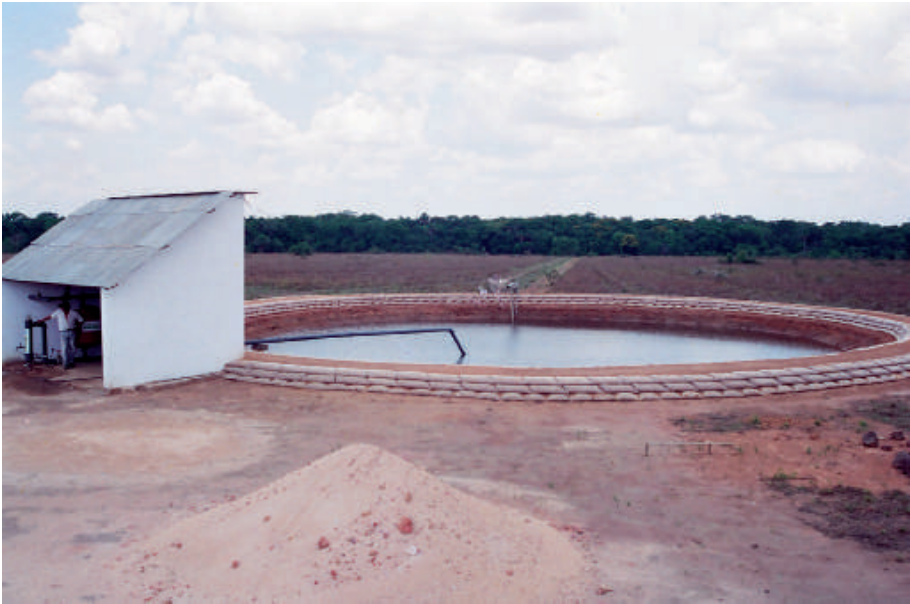
Dam from gabions made by soil-cement in GAVIOTAS caribbean pine nursery
