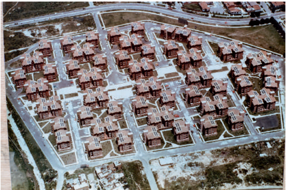
GAVIOTAS solar installation of water heaters in the Nueva Villa de Aburrá urbanization in Medellín city
