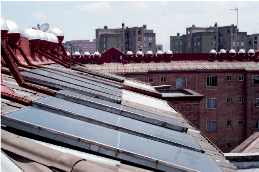
GAVIOTAS solar heaters installation for 1.100 apartments
