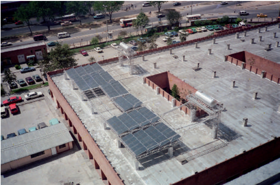
GAVIOTAS solar water heaters installation in Mederi Hospital Bogota
