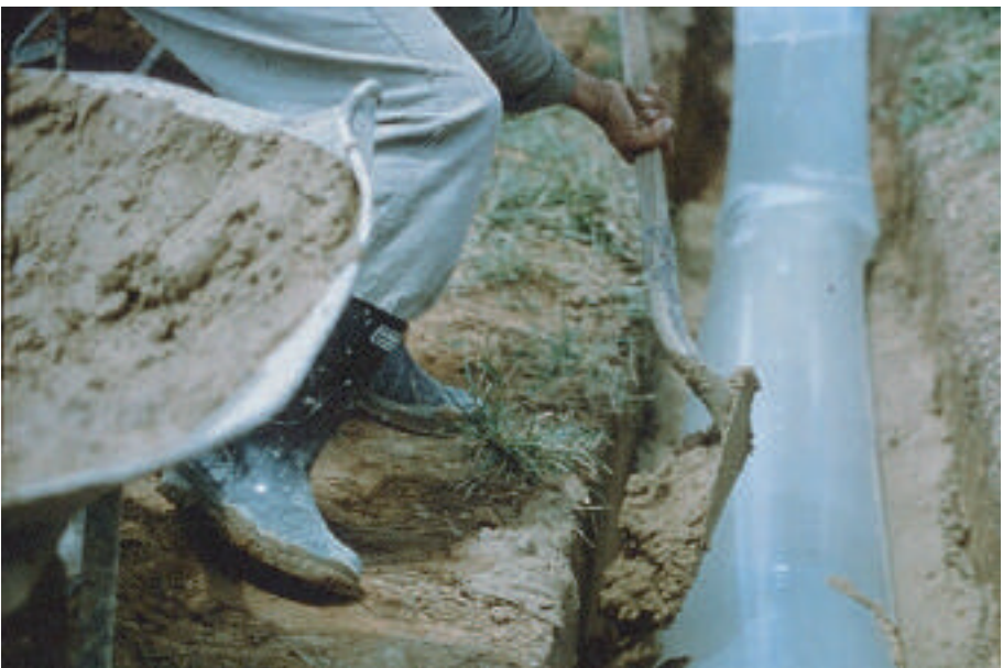
GAVIOTAS type pipe manufacture
