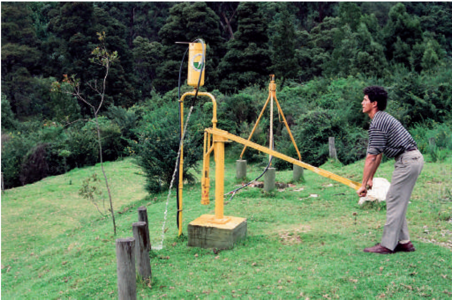
GAVIOTAS remote control pump for extracting water
