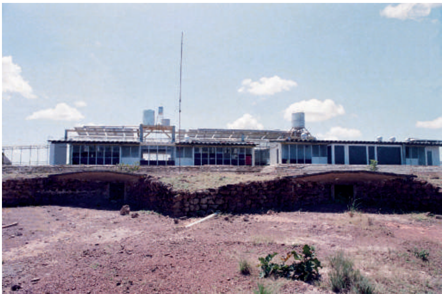
underground ducts for venting the natural tropical water bottling in GAVIOTAS
