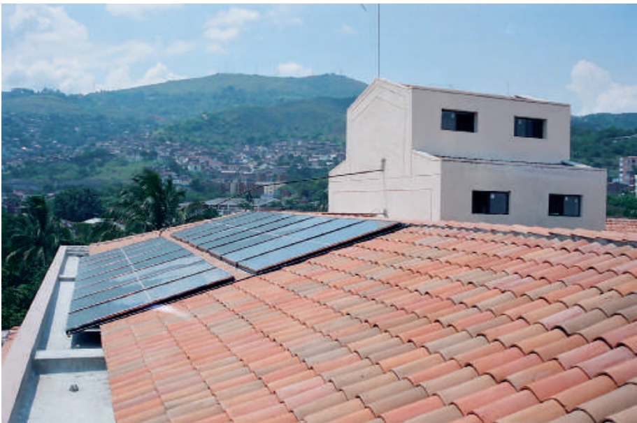
GAVIOTAS solar heaters installation in a religious community, Cali City
