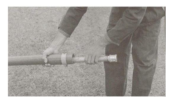
Held tight the sleeve using the braces, tie the galvanized pipe with a rope for avoiding it to fall into the sleeve and screw it in the bottom of the head.
