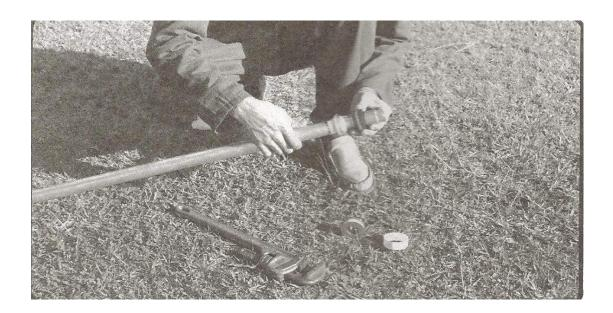
Do not let the leather plunger to become wet before you have introduced the galvanized pipe inside the PVC sleeve.
