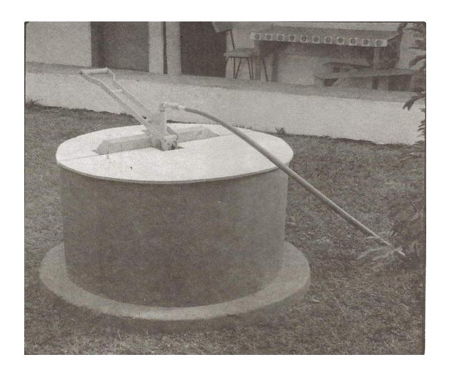
It is necessary to cover the well with a lid so the water could be protected from the solar rays, and to prevent it from dirt and other objects, do not allow animals to sleep on the well.
