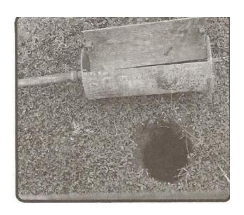
16 cm diameter drilled hole and depth 11 ms before being coated.
