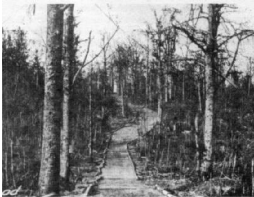
Part of an 1,800 foot plank road built through a sea of mud. Credit: battalion archives
