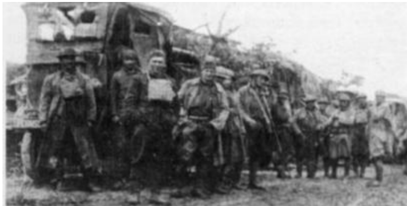
The engineers waiting along the roadside to attempt to force a pontoon bridges crossing of the Vesle River Credit: battalion archives
