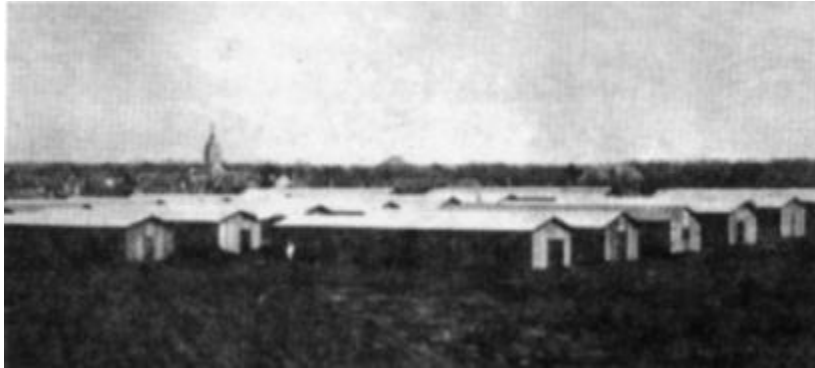
A complete hospital built by the 107 th in Chateauvillain, France Credit: battalion archives
