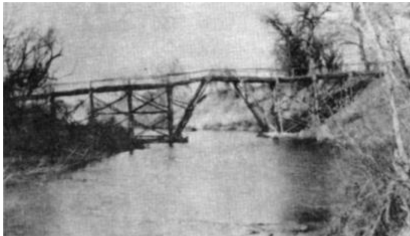
One of the many training bridges built by the 107 th in Texas Credit: battalion archives
