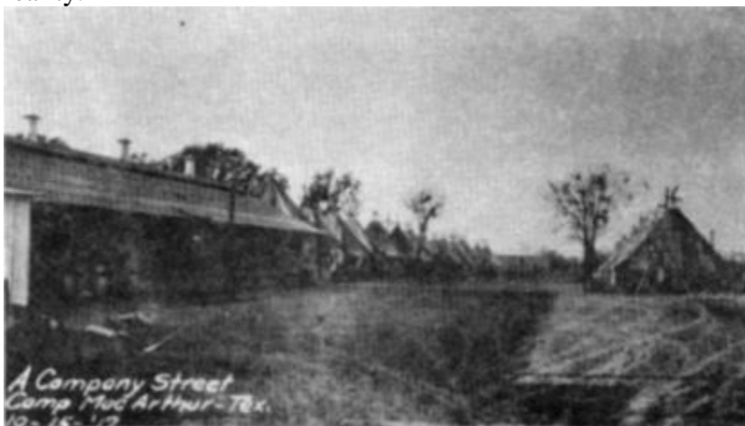
Company A's company street at Camp MacArthur, Texas Credit: battalion archives
