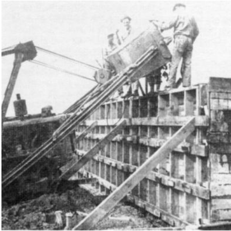
Company B pouring concrete for a training pillbox.
