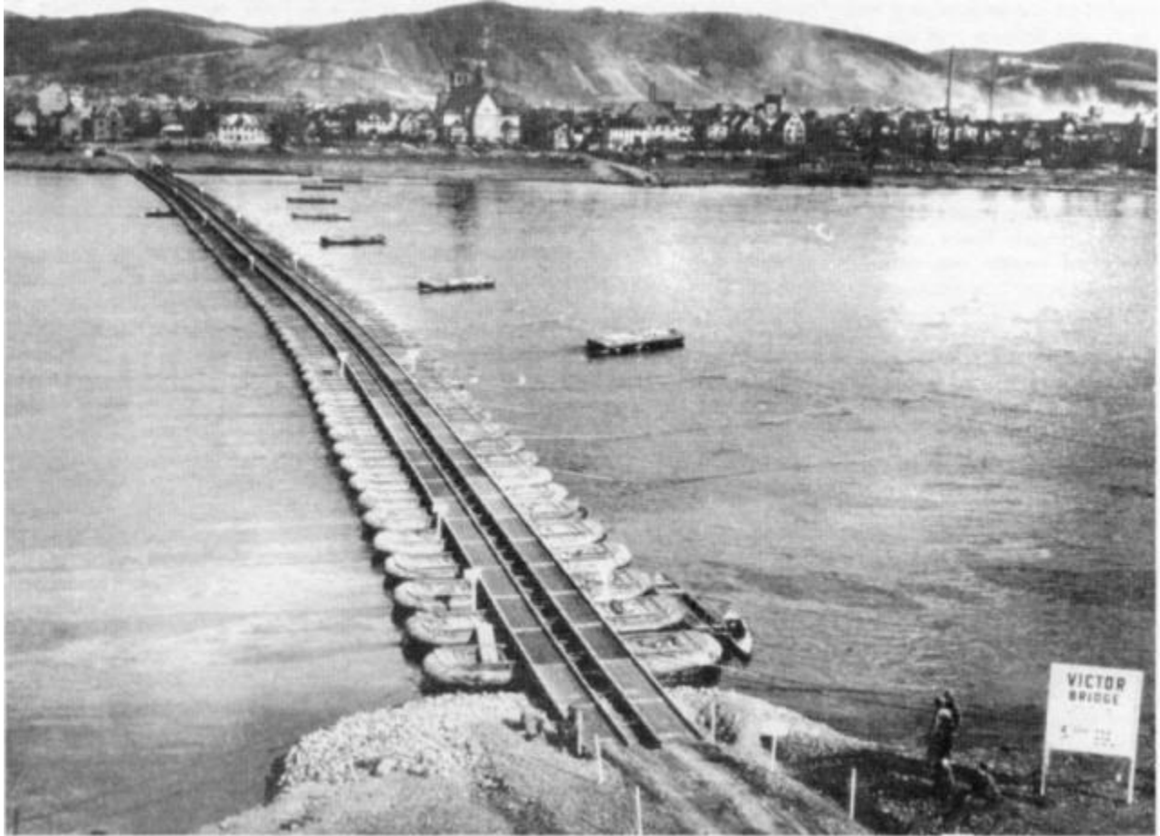
To bridge the Rhine River the Battalion built the 1,730 foot Victor Bridge and set a record the still stands for the longest tactical floating Bridge ever constructed. Credit: battalion archives
