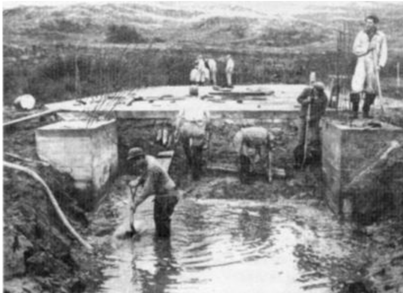
Constructing the assault training center near Slapton Sands. Credit: battalion archives
