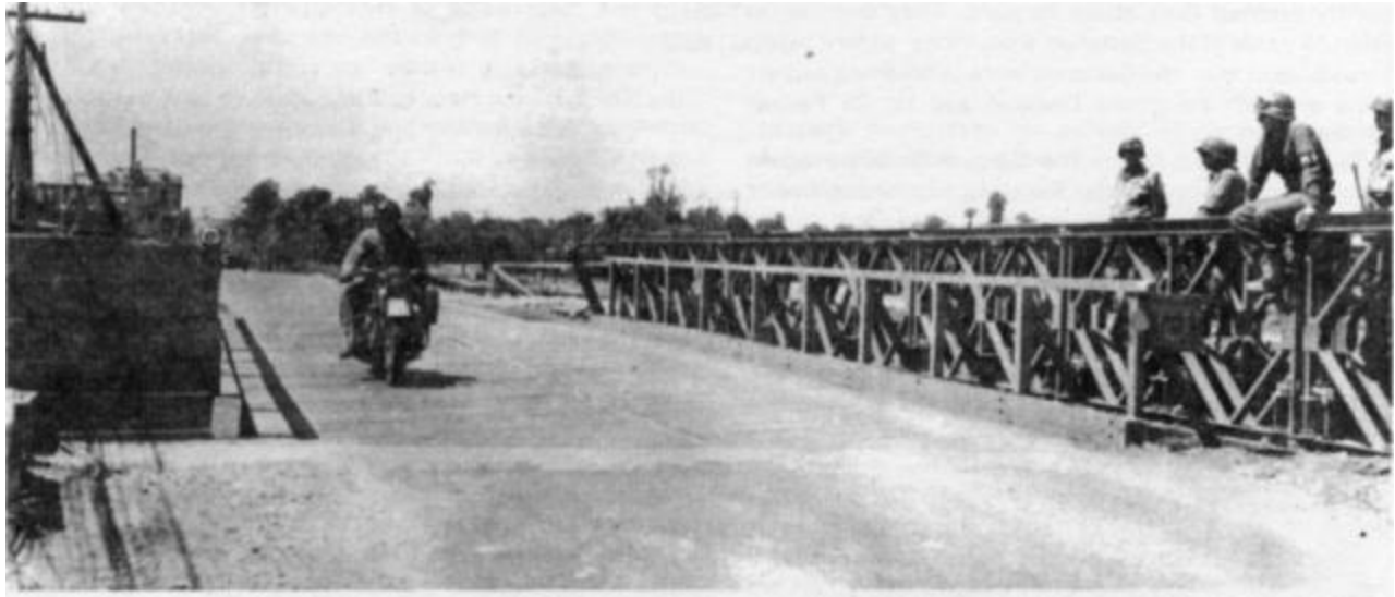
A replacement timber trestle bridge built next to a Bailey Bridge.
