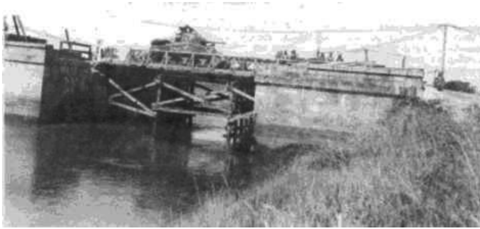
A Sherman tank crossing a timber trestle bridge built by the Battalion. Credit: national archives
