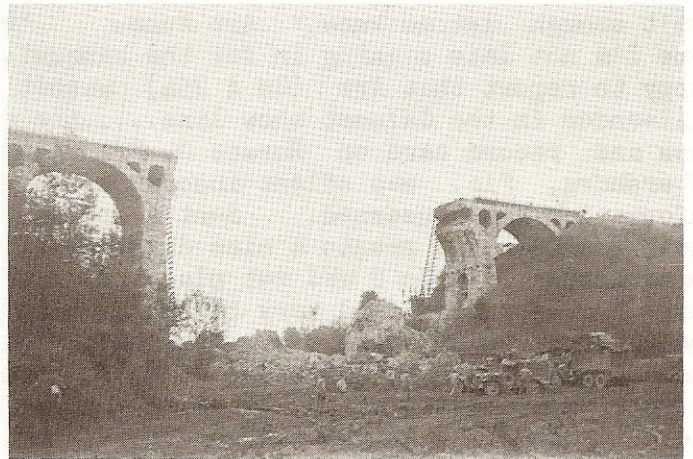
An example of railroad demolitions (Belgium) (continued next page)
