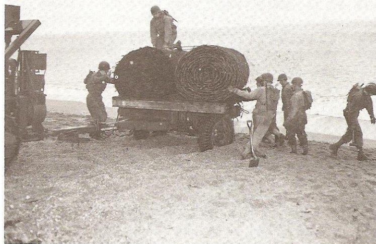
Unidentified Co A 254 soldiers with strip packs manually turning turntable built on trailer in position for dropping mats during hasty beach road experiments. SLAPTON SANDS, DEVONSHIRE, ENGLAND - 3 Feb 44
