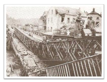
The bridge constructed by the 254<sup>th</sup> in Gemünd after it collapsed. (The remains of the concrete bridge it replaced can be seen under their Bailey bridge.)
