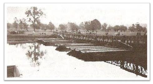
Floating Bailey bridge under construction at Wallingford
