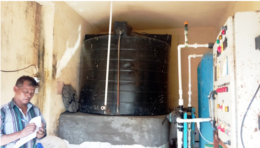
After water tank base height
