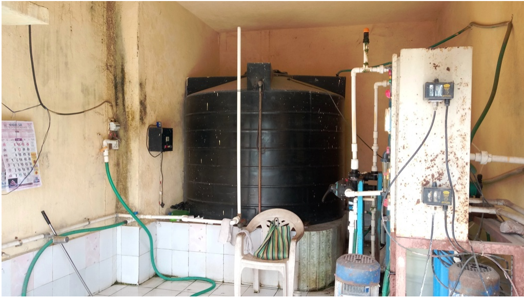
Before water tank base height
