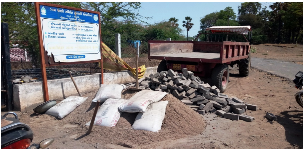
During the work of water tank height and color work
