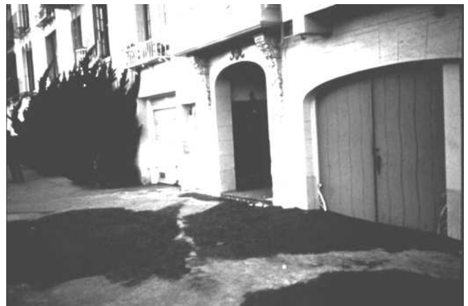
Figure 40 - Loma Prieta Earthquake, October 17, 1989. Lateral spreading, liquefaction and sand boils caused extensive damage in the Marina District of San Francisco, about 60 miles away from the epicenter.
