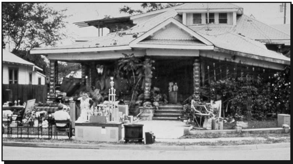
Damage from magnitude 6.7 earthquake
