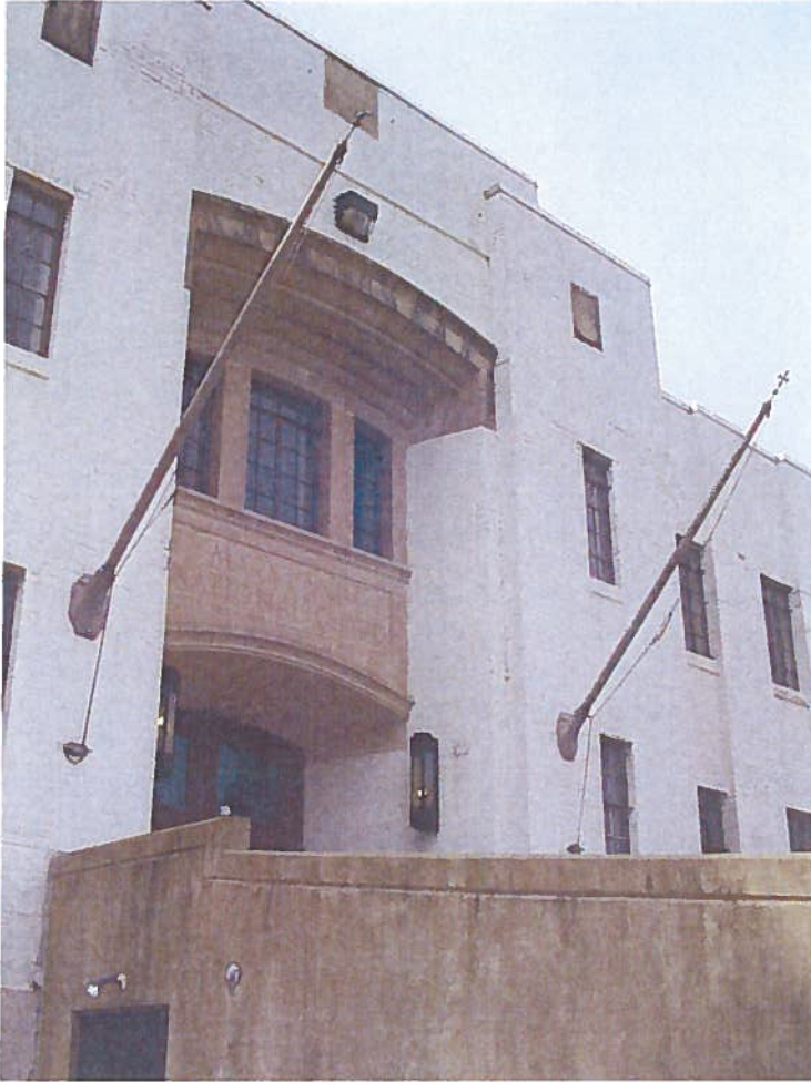
Photo 1 – View of the front entrance to the Chestertown Armory building located at 509 Cross Street in Chestertown, Maryland.
