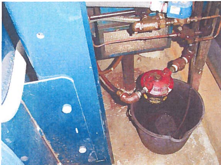
Photo 20 – Close-up view of the boiler unit for the Chestertown Armory building located at 509 Cross Street in Chestertown, Maryland.
