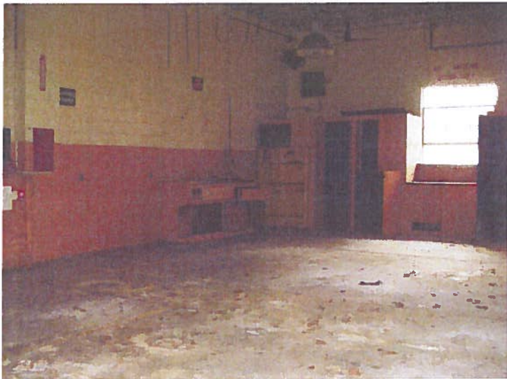
Photo 24 – Inside view of the maintenance garage portion of the Chestertown Armory building located at 509 Cross Street in Chestertown, Maryland.
