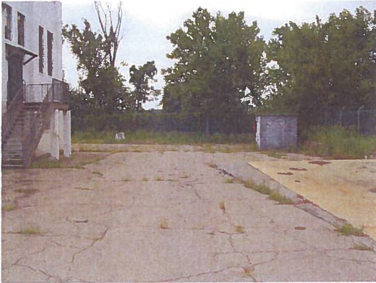
Photo 6 – View from the west showing the Chestertown Armory property on the south side of the armory building located at 509 Cross Street in Chestertown, Maryland.
