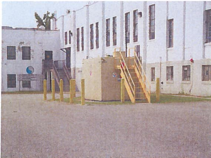
Photo 2 – View from the northwest showing the 6,000-gallon AST located at the northeast corner of the Chestertown Armory building located at 509 Cross Street in Chestertown, Maryland.
