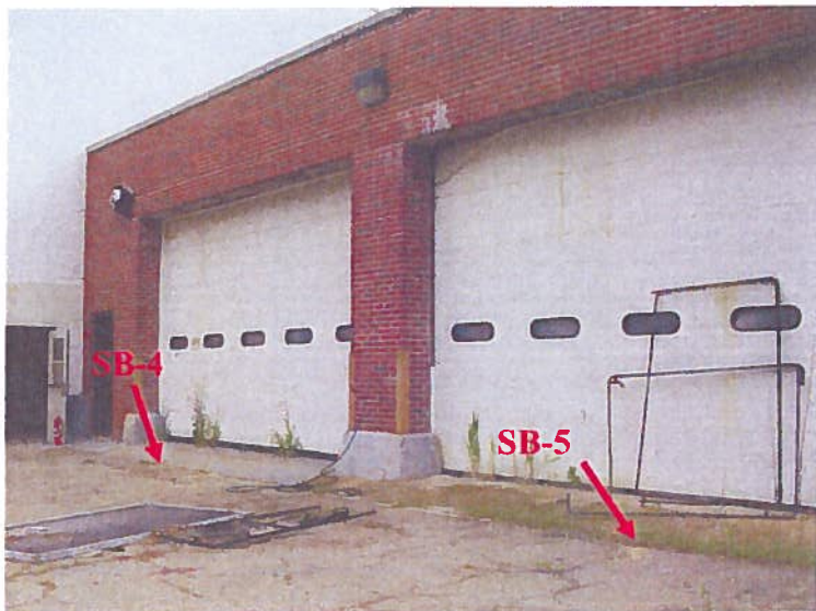
Photo 10 - View from the southeast showing the maintenance garage portion of the Chestertown Armory building located at 509 Cross Street in Chestertown, Maryland. Soil borings SB-4 and SB-5 are identified in the photo.
