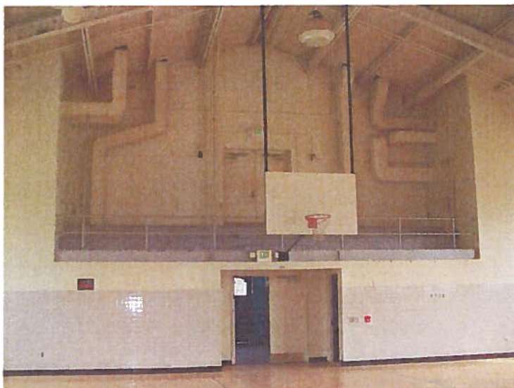
Photo 13 – Inside view of the main portion of the Chestertown Armory building located at 509 Cross Street in Chestertown, Maryland.
