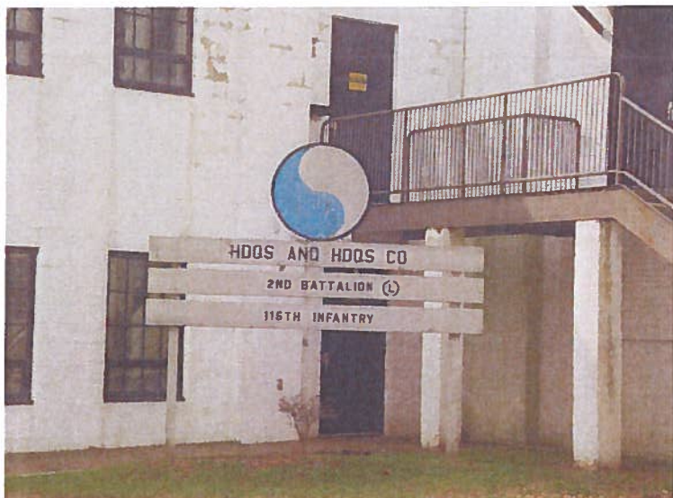
Photo 5 – View from the west of the Chestertown Armory building located at 509 Cross Street in Chestertown, Maryland.
