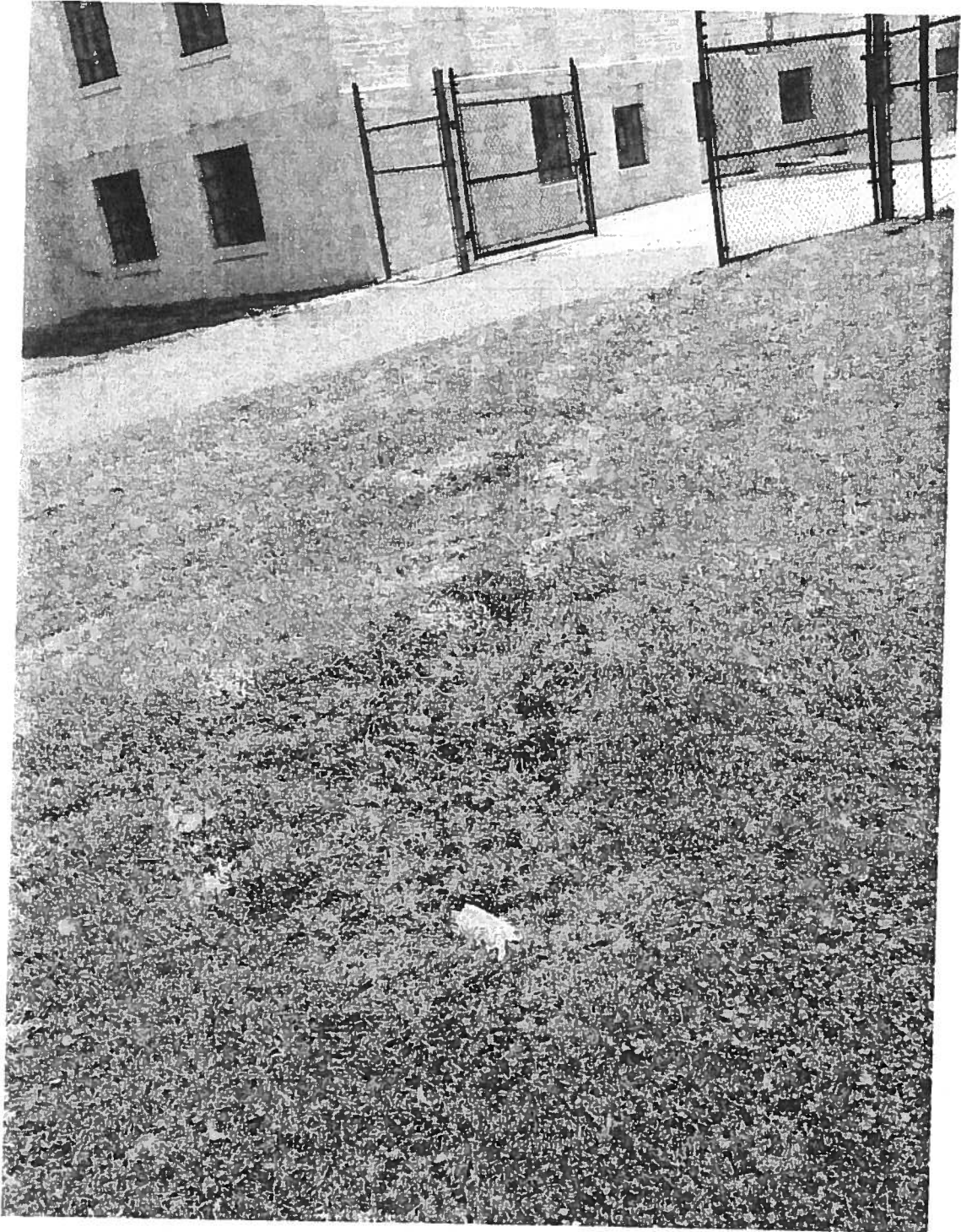
Rut from Hurricane Isabel Unit would like some fill to fix rut as a self- help effort.
