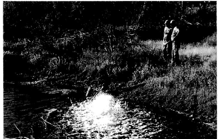
Dave & Tom manage the water discharge into the coffer dam
