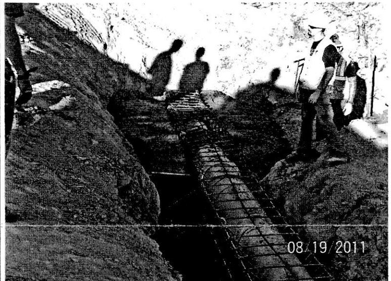
Encasing the drain pipe in concrete begins.
