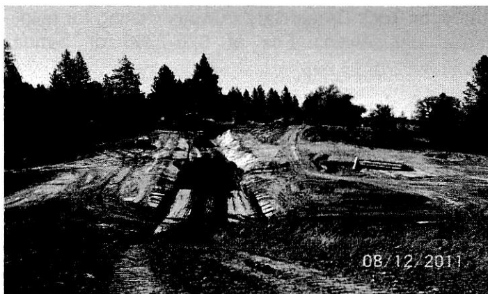
Cutting the "keyway"
