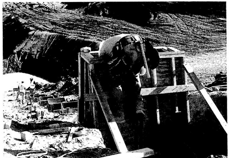
Working on Slide Gate Support
